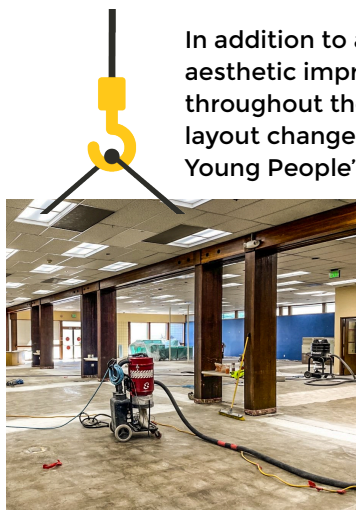
Sparks is ready for new floors!
