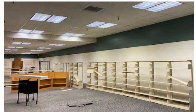
With shelving off the walls, painting has begun!
